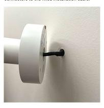
5. Carefully push the cable back into the hole. This is easier if the hole is larger than 16mm or there is a wall cavity.
